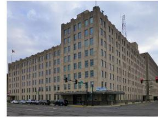
(c) Office Building
