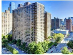
(b) Apartment Building
